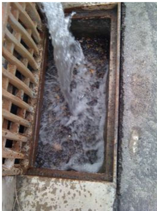
Xeripave filtration tray in catch basin.
